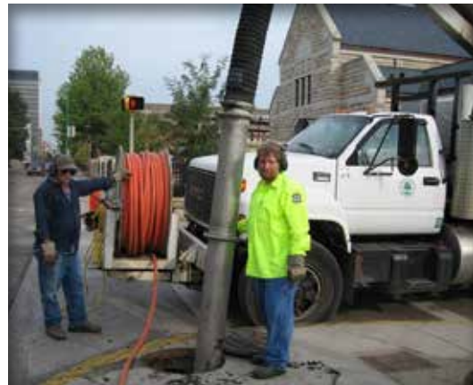
Figure 8-1.1 Maintenance of City's Storm Drain
