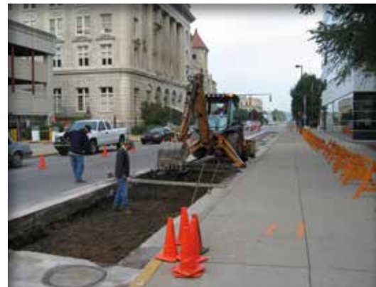
Figure 8-1.2 City Field Crew doing Street Maintenance
