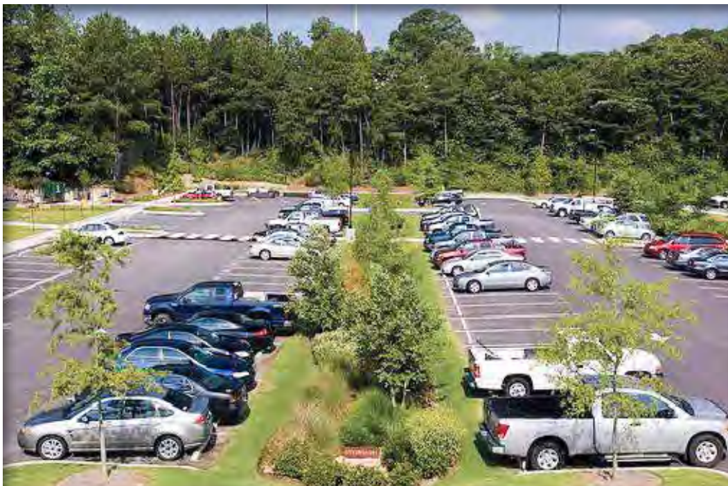
Figure 3-4.11 Parking lot Bioretention Garden
