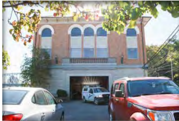
Figure 3-4.13 Building in Charleston with a Reduced Impervious Footprint Due to Parking Beneath Building
