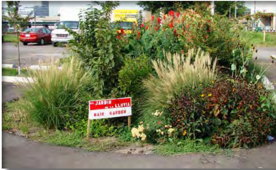
Figure 3-4.18 Parking lot collection Rain Garden
