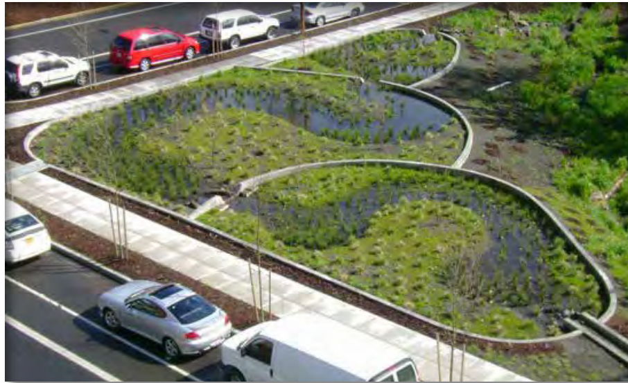
Figure 3-4-15 Example of Detention Garden use to slow water discharge
