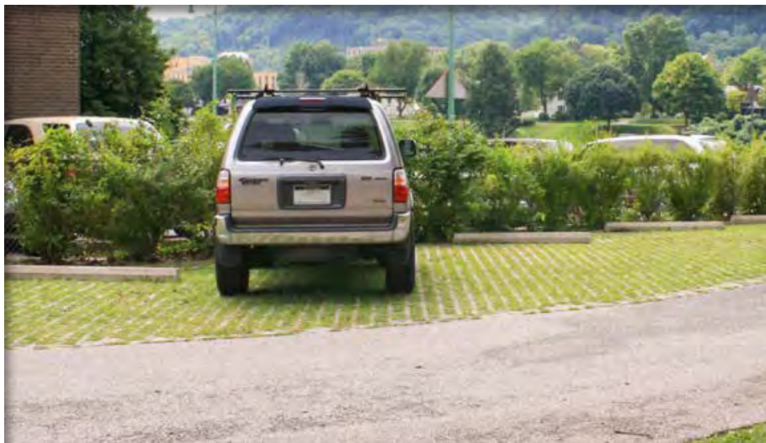
Figure 3-4.12 Parking area paved with turf block paver
