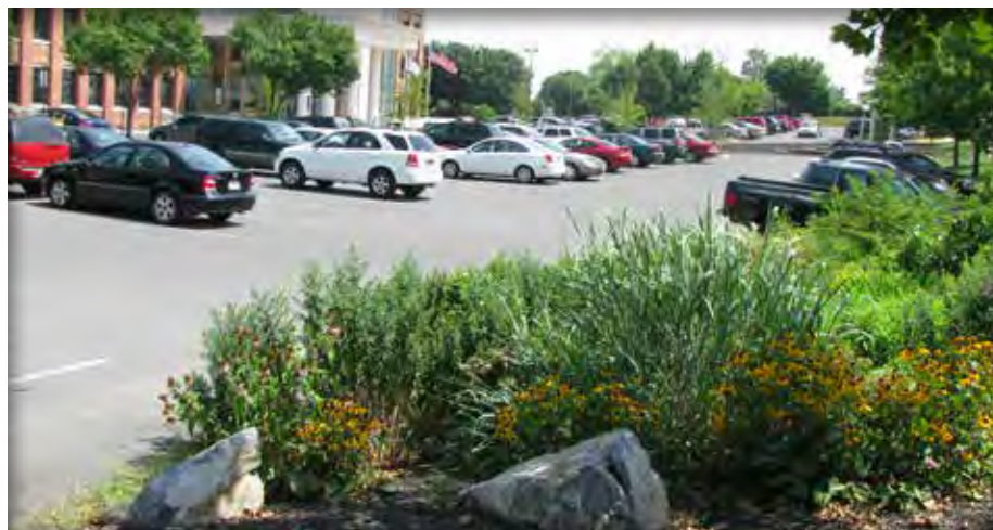
Figure 3-4.16 Rain Garden at Berkeley County Courthouse
