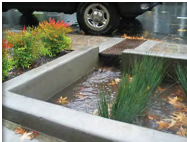
Figure 3-5.3 Four (4) Inch Curb Exposure
