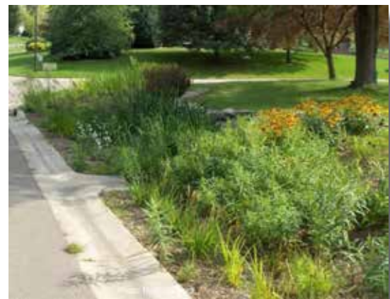
Figure 1-2.5 Roadside detention area
