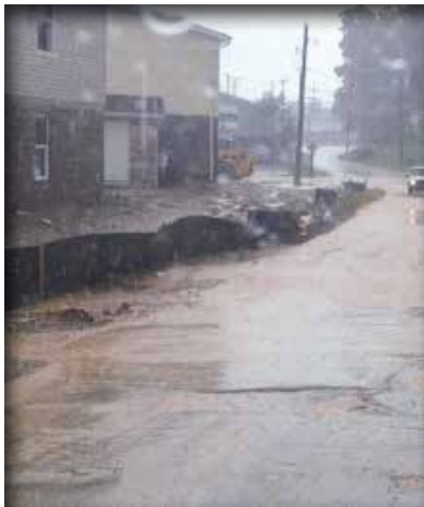
Figure 1-2.4 Erosion from jobsite
